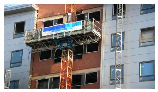
Figure 14 A mast climbing work platform
