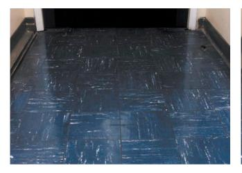
Figure 48e Asbestos-containing vinyl floor tiles
