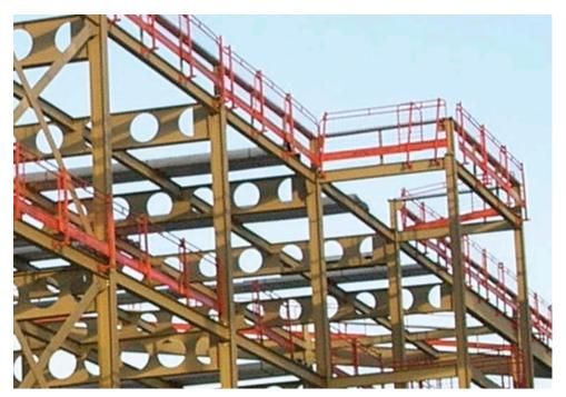
Figure 28 Edge protection installed with the steelwork
