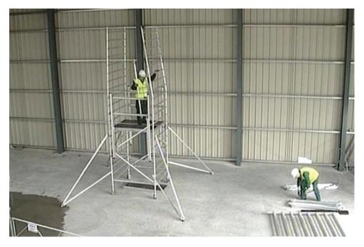
Figure 11 Advanced guard rails
