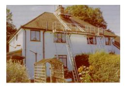
Figure 25 Proprietary access system for roof-work
