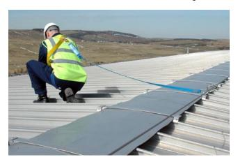
Figure 16 A work-restraint harness
