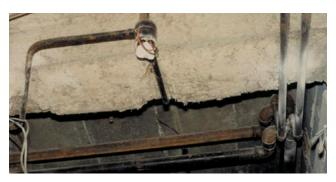
Figure 48b Poorly tamped sprayed chrysotile fireproofing on a structural steel beam holding up a concrete floor, showing some overspray onto the concrete and damage by electrical work
