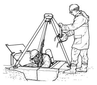
**Figure 51** A worker wearing full breathing apparatus is also wearing a harness and lanyard connected to a winch so that he can be hauled to the surface in an emergency without others having to enter the manhole to rescue him
