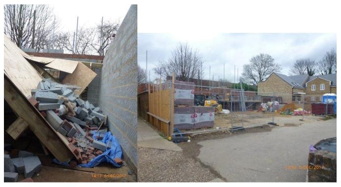
An investigation by the Health and Safety Executive (HSE) found that the Principal Contractor, S McMurray Ltd, had failed to safely install joist hangers correctly. There was no other structural support arrangement in place, such as propping the first floor from underneath. The floor was also overloaded with blockwork.
